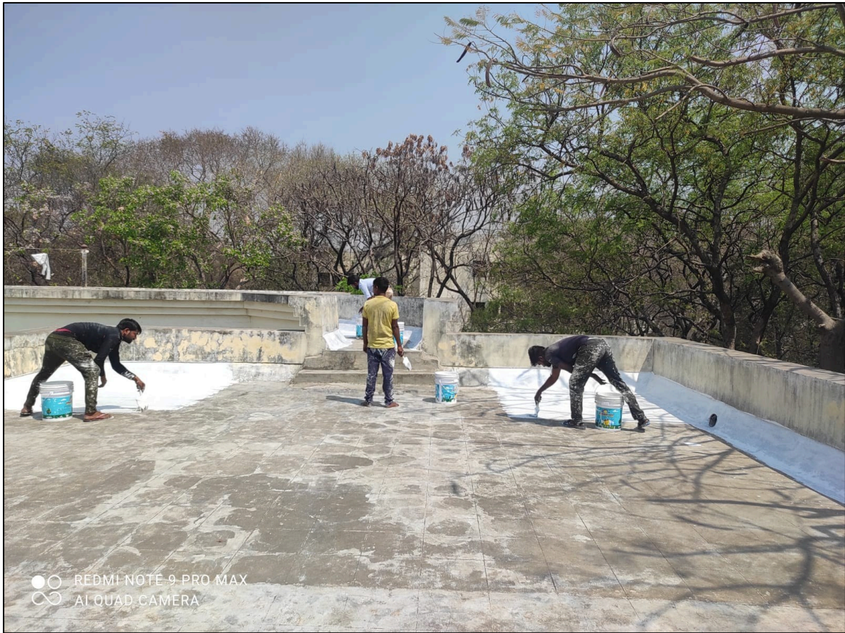
Figure 9 Cool Roof Painting During Progression
