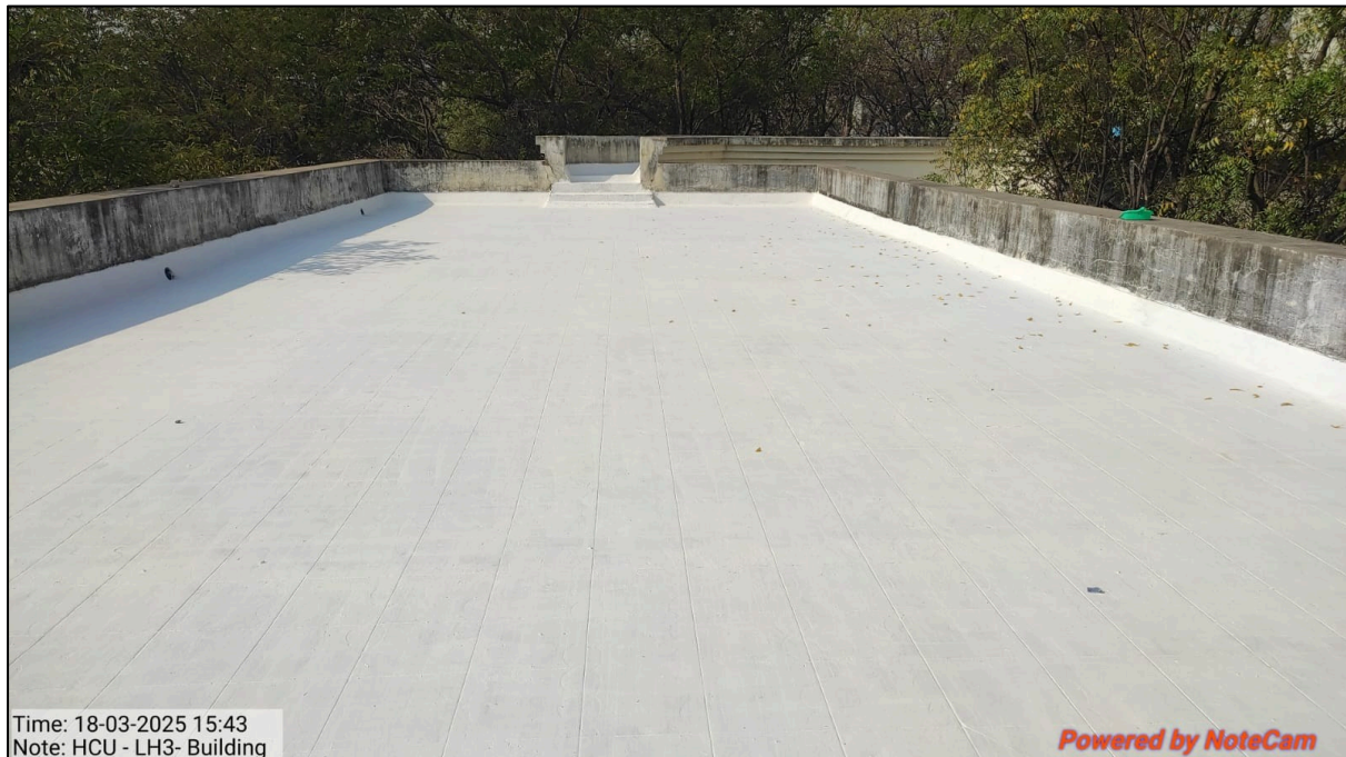
Figure 10 Cool Roof Painting After Completion
