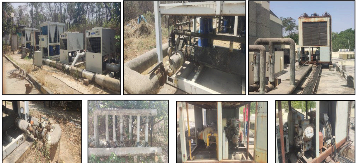
Figure 2 Condition of Existing Chiller Systems
